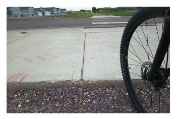
FIGURE 3.7 The unpaved path at the intersection of W Willow Street with Honeysuckle Drive has a vertical trip hazard where the unpaved and paved surfaces meet. This can be corrected by adding material to meet the level of the concrete surface.
