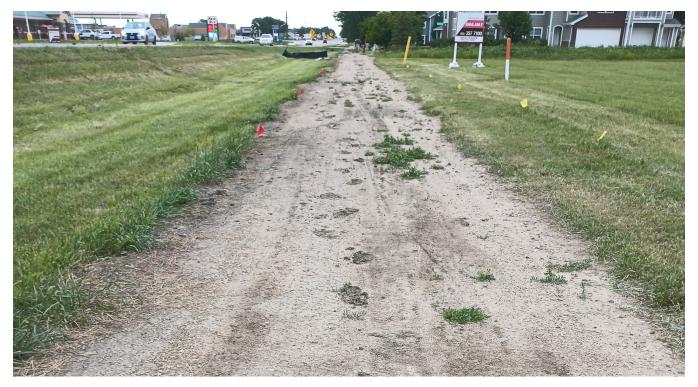
FIGURE 3.6 Footstep and bicycle wheel indentations can be seen on this segment of unpaved trail along Willow Street.
