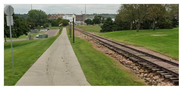
FIGURE 4.14 An example of a rail-with-trail facility at Falls Park in Sioux Falls. Credit: Google
