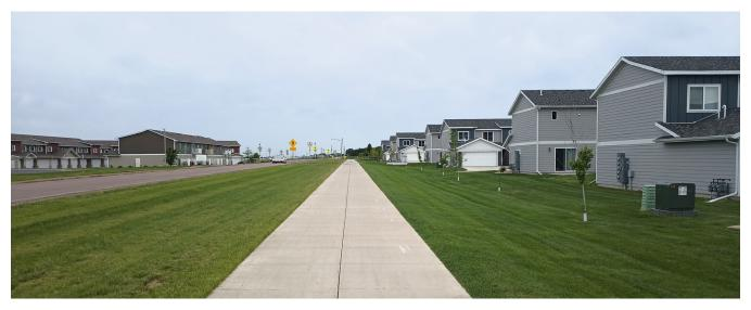
FIGURE 3.4 The Willow Street trail along the north side of the road is 10' wide and concrete.
