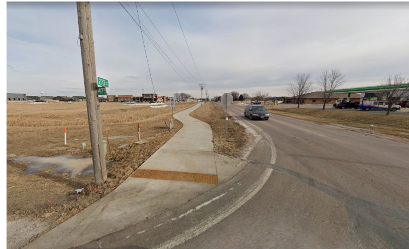
Sidepath at Willow Street and Cliff Avenue
