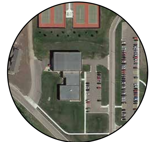
2 ALTERNATIVE HIGH SCHOOL BUILDING
