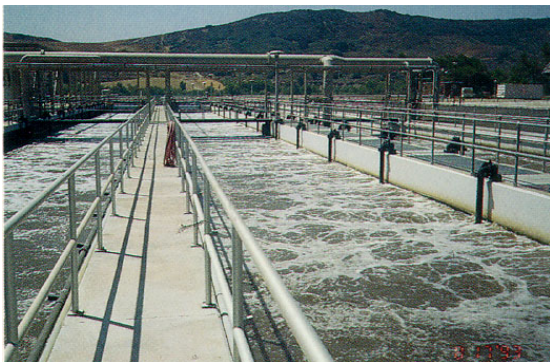
Plug flow activated sludge system
