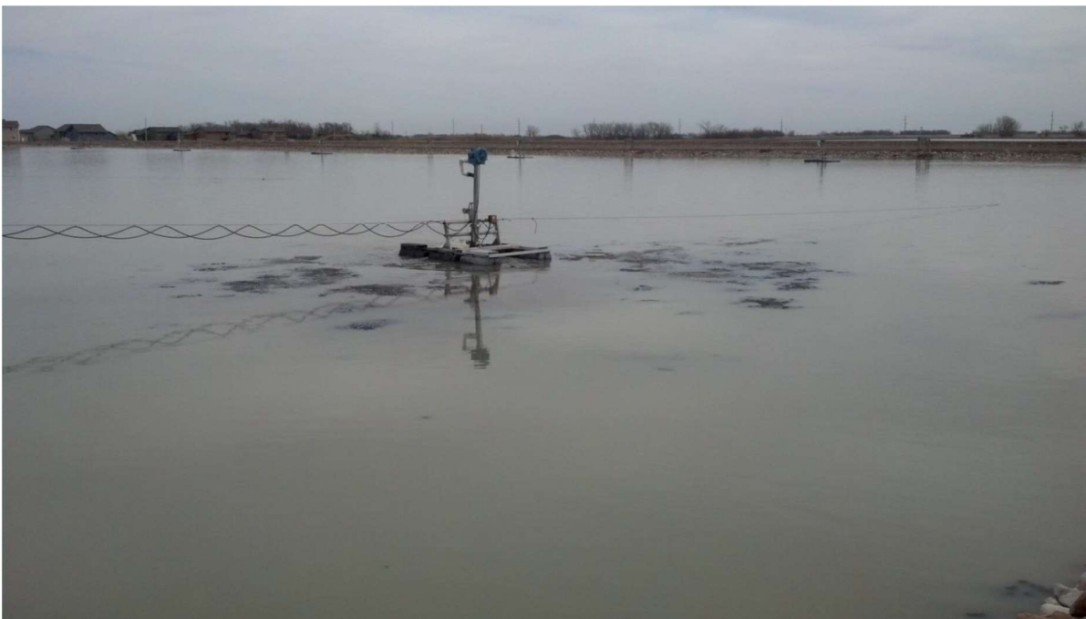
Figure 10 Sludge Build-up
