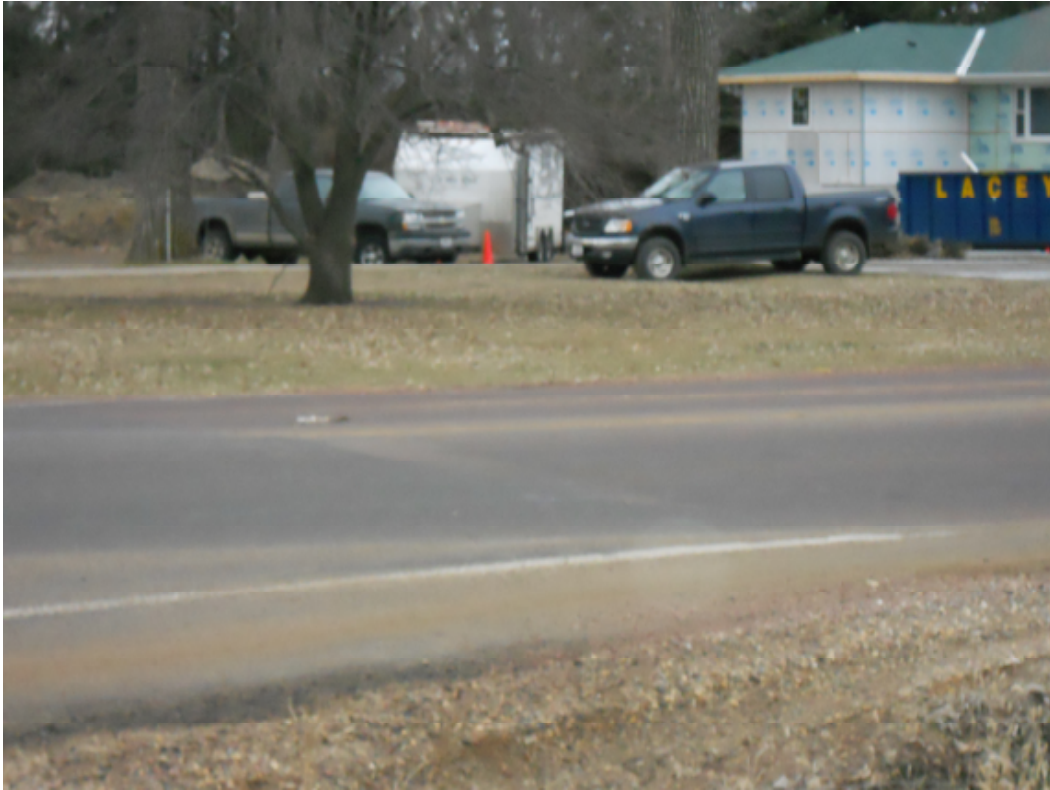
Pavement on Cliff Ave. North of HWY 106
