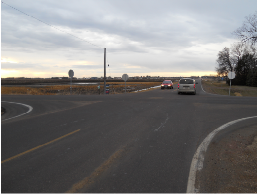
HWY 106 and Cliff Ave. (Looking West)
