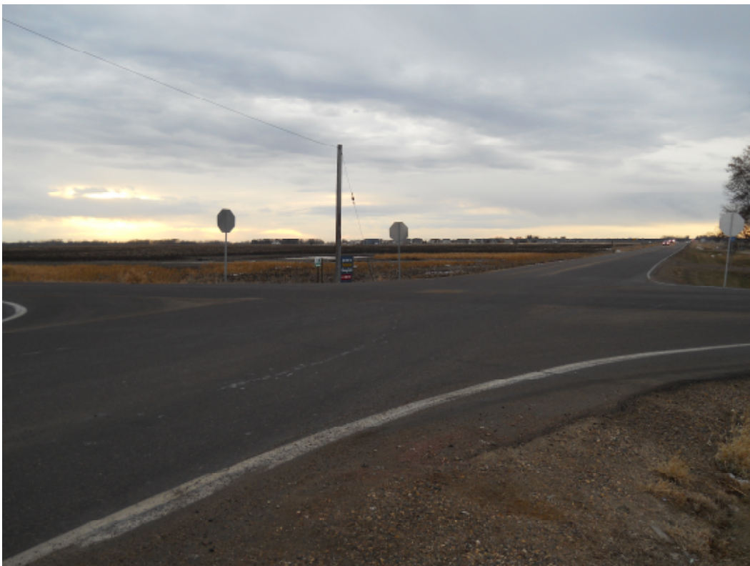
HWY 106 and Cliff Ave. (Looking SW)
