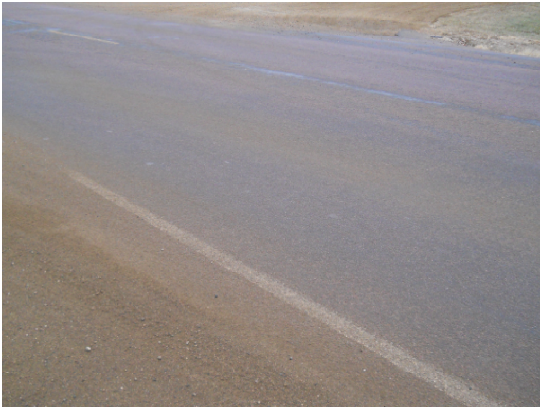
Pavement on Minnesota Ave. at 272 nd Street
