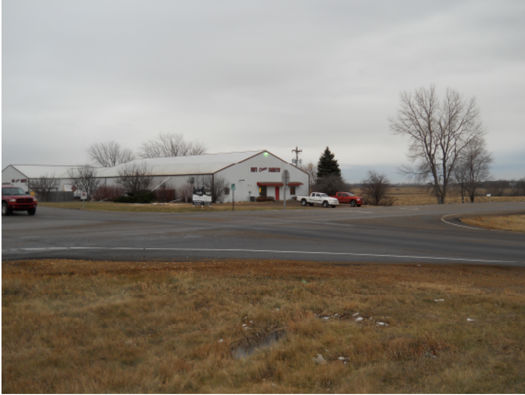
Willow Street and Minnesota Ave. (Looking SE)
