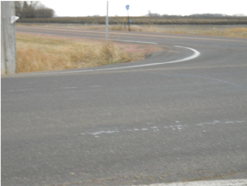
Pavement on HWY 106 East of Cliff Ave.
