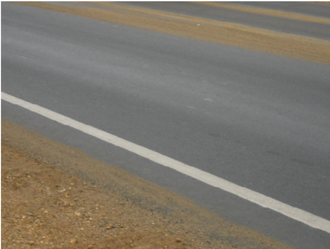
Pavement on Willow Street West of Minnesota Ave.
