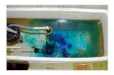
**Step 7.** To check a toilet for a leak: Flush the toilet and while the reservoir is still filling, add 2 or 3 drops of food coloring to the water in the reservoir.
