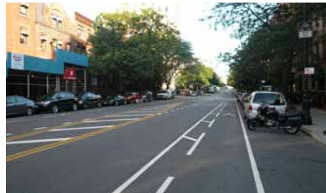
Figure 7.7. Bike Lane Pavement Markings. Source: AASHTO 2010
