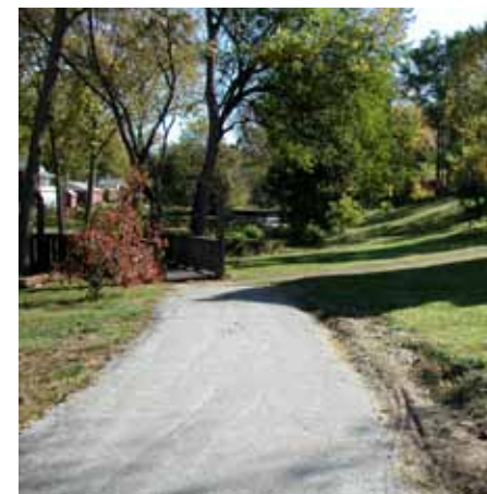
Interim Surfaces. Lower-cost surfaces can establish a pattern of trail use if full funding is unavailable for a period of time.
