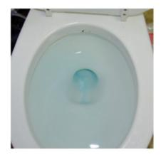
Wait 15-30 minutes. If the water in the bowl changes colors, the flapper valve needs to be replaced.
