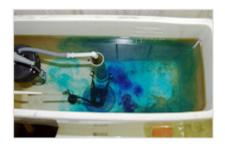
**Step 7.** To check a toilet for a leak : Flush the toilet and while the reservoir is still filling, add 2 or 3 drops of food coloring to the water in the reservoir.
